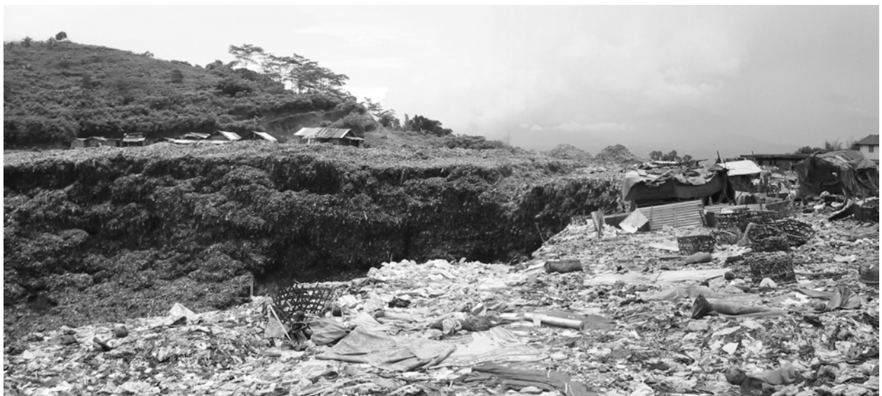
Figure 2: Slope crest with civil constructions clustering on the right and in the back
